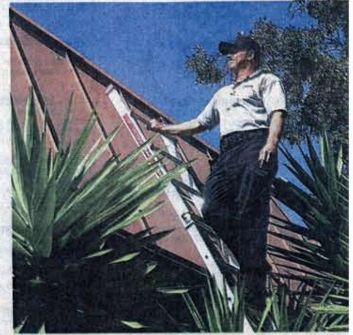
Sean Blasius, owner of Best Property Inspections, takes a look at the roof line of this Carlsbad building. Christine Davis
